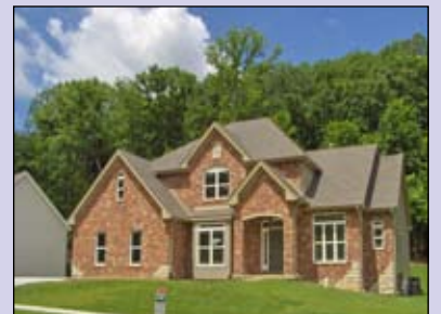
773 SOUTHERN HILLS DRIVE Eureka New Construction • $589,900
